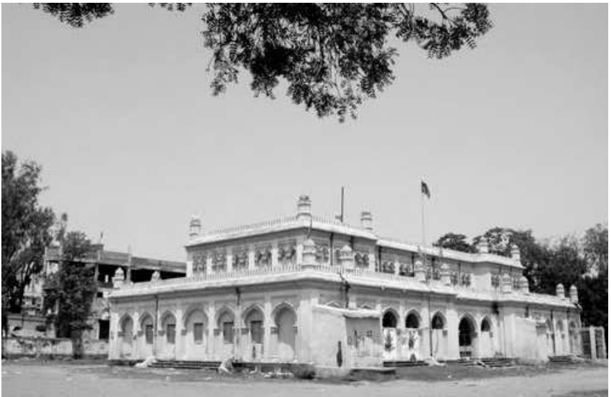
▲ A VIEW OF TOWN HALL IN SAMBALPUR
