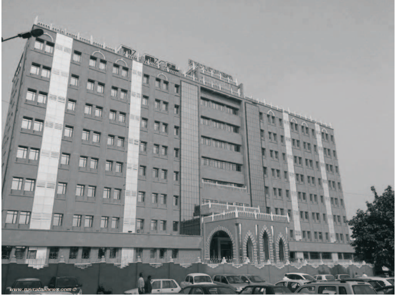
▲ BUILDING OF ODISHA HIGH COURT
