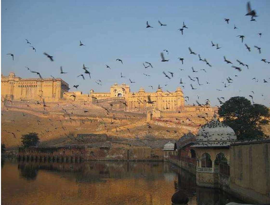
Rajasthan ke Durg in Hindi
